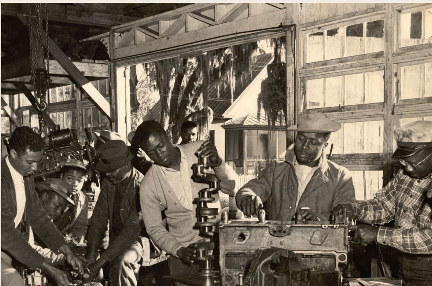
Circa 1950s. Auto Mechanics class – Savannah State College Students in Savannah State College's auto mechanics class overhaul an engine, instructed by Professor Leroy Brown, Image courtesy of Savannah State University (GA) Asa H. Gordon Library Special Collections.
